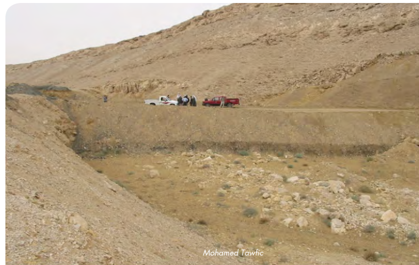
Road Construction, Obstructing Flash Flood Reaching the Bedouin in Sinai
