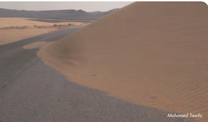
The Main Road Of El Maghara Area Covered With Moving Sand Mohamed Tawfic
