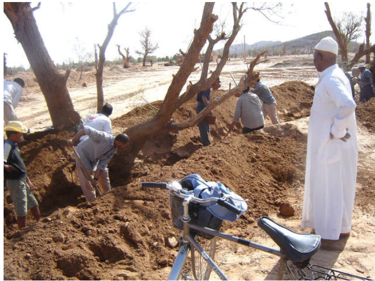
Photo 19: Cleaning out 'Souaguis' in the oasis of Ferkla
